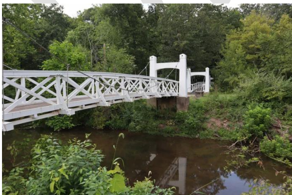
Pedestrian Foot bridge-Lenape Park
