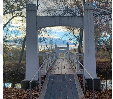
1937 Roebling Style Twin Foot Bridges - Lenape Park
